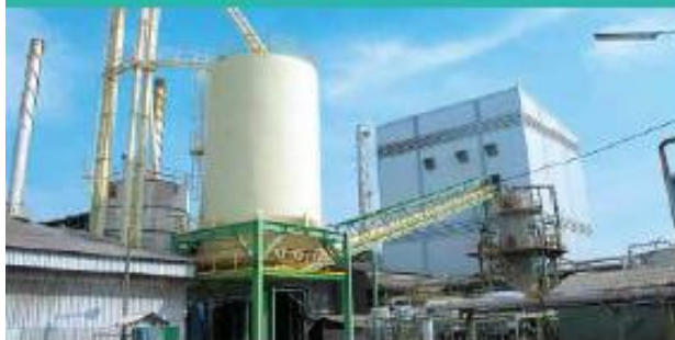
Biomass Boiler (Thailand)/ Fuji Foods Corporation
