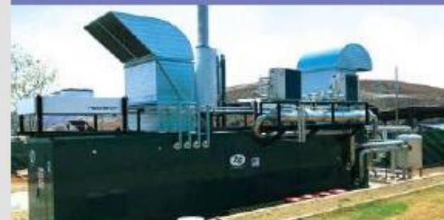
Power Generation with Methane Gas Recovery System (Mexico)/ NTT Data Institute Consulting Inc.
