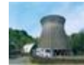
Geothermal power generation
