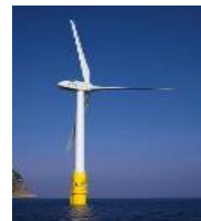
Wind power generation
