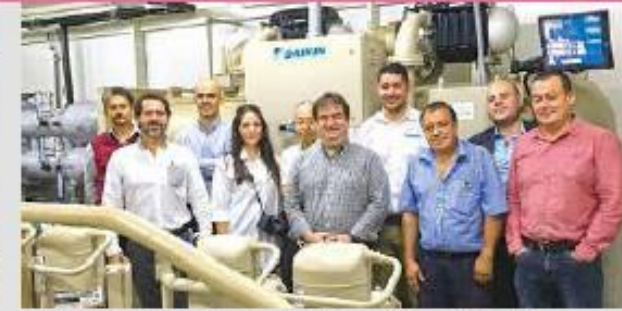
Chiller and Heat Recovery System (Costa Rica)/ NTT Data Institute Consulting Inc.
