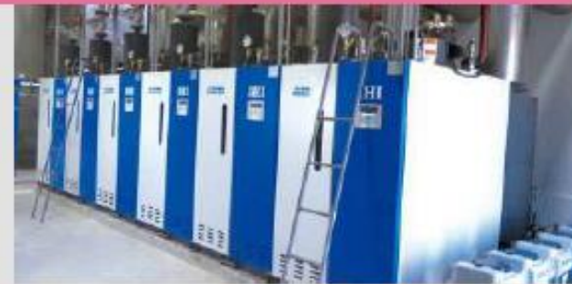
Once-through Boiler (Myanmar)/ Acecook Co., Ltd.
